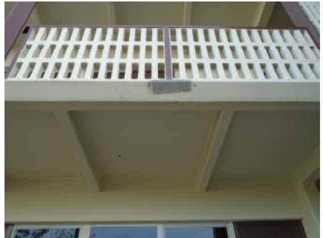
Fig 9. Existing recent spawled concrete repair
