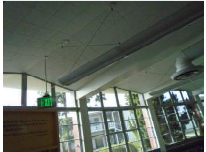
Fig 2. Folded plate roof from interior
