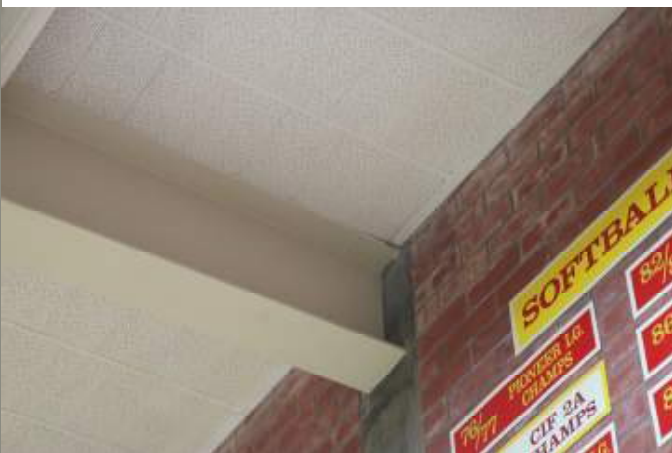
Fig 5. TSG connection at concrete column in gym
