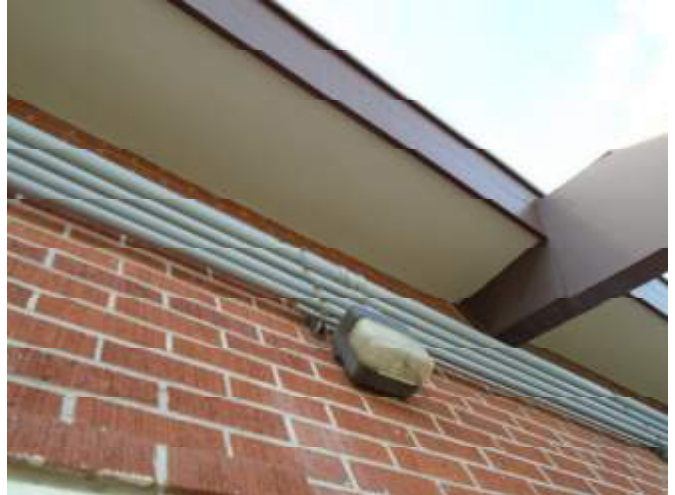
Fig 2. Masonry side wall & glue lam arch with sheet metal protection
