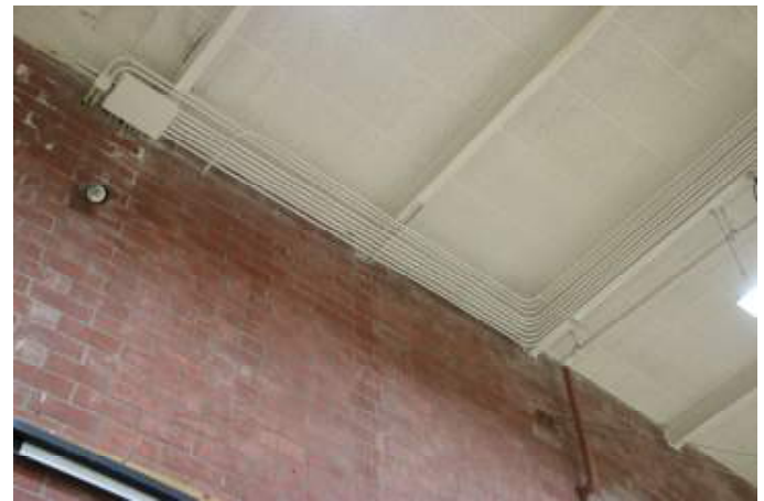
Fig 4. Purlins at masonry wall in gym
