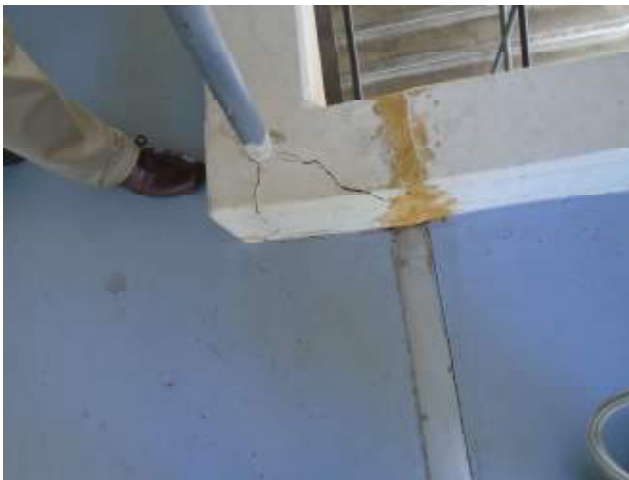
Fig 8. Cracked concrete at guard rail
