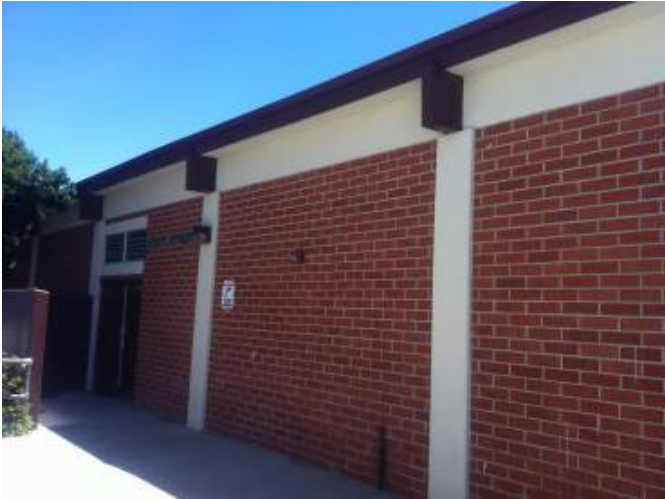
Fig 1. Exterior masonry wall with concrete piers
