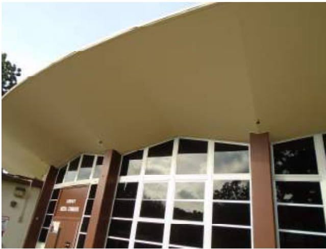
Fig 1. Folded plate roof and support piers from exterior
