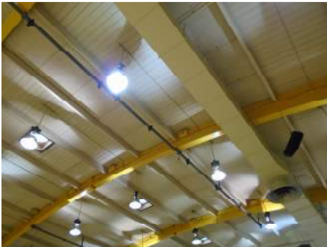
Fig 3. Glue lam roof support arches inside the gym
