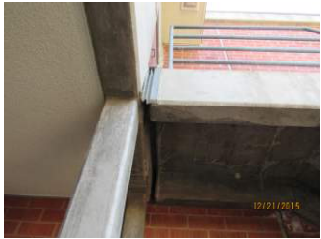
Fig 4. Structural separation at circulation
