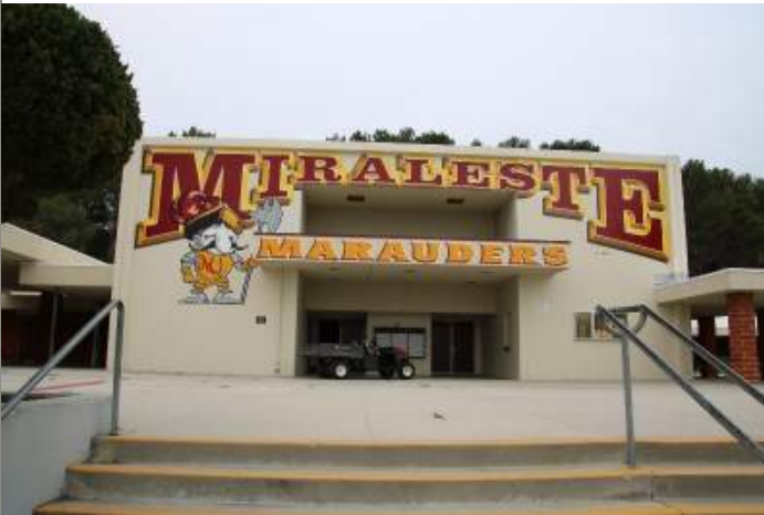
Fig 1. Precast wall panels at front of MP room
