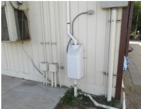
Photo #35: Radon Gas Detector And Evacuation System
