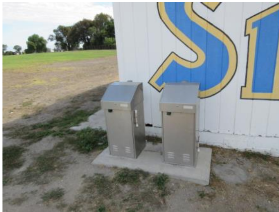
Photo #27: Irrigation Controllers
