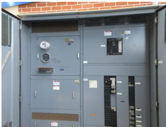
Photo #23: Main Electric Panel
