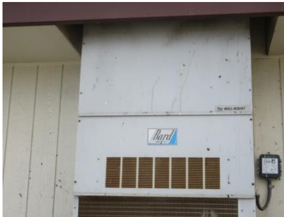
Photo #21: Wall Mounted HVAC Package Unit
