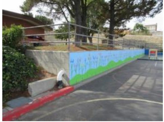
Photo #14: Retaining wall
