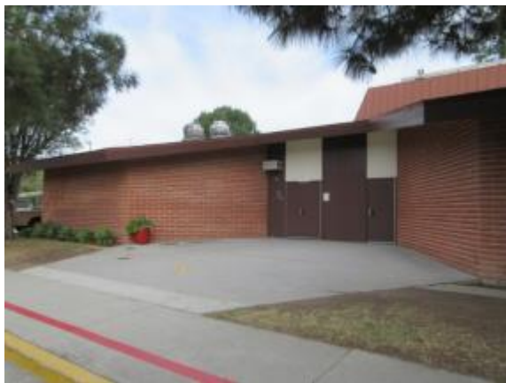
Photo #3: Classroom rear elevation
