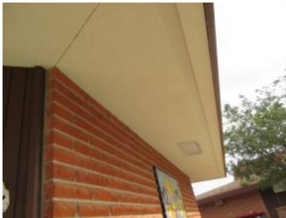
Photo #21: Soffit structure
