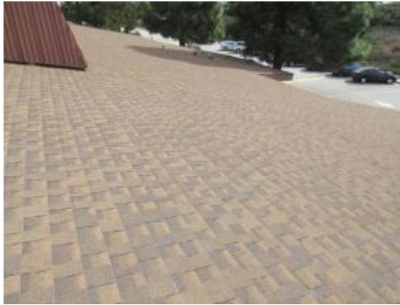
Photo #19: Permanent building roof
