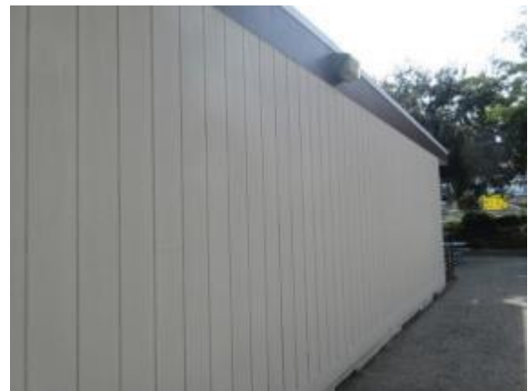
Photo #6: Modular classroom side elevation
