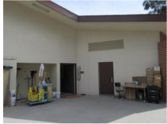
Photo #2: Multipurpose room west elevation
