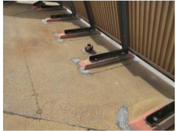
Photo #20: Roof at equipment well
