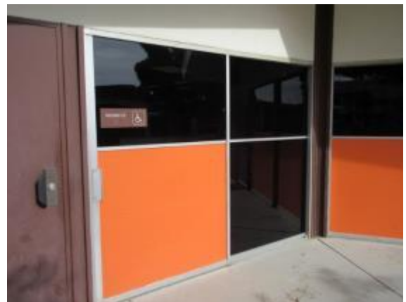
Photo #24: Sliding door at classroom
