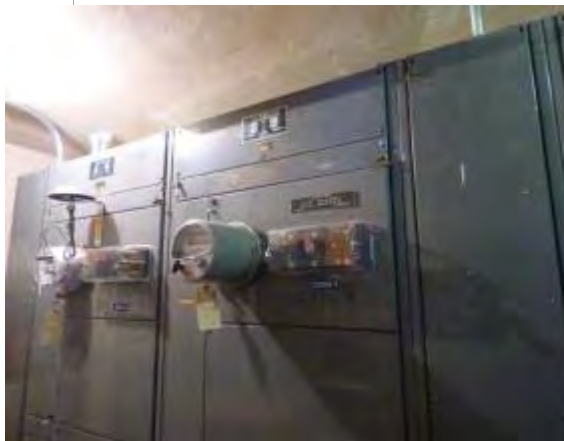
Photo #47: Main electrical switch gear at building #100 electrical room
