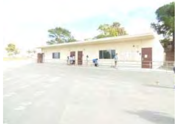
Photo #54: Locker room portable buildings.
