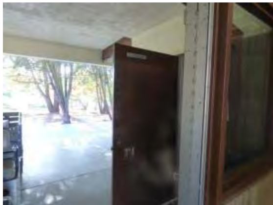
Photo #27: Finishes around classroom buildings
