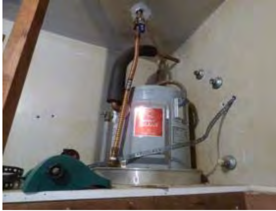
Photo #43: Water heater at restroom mechanical room
