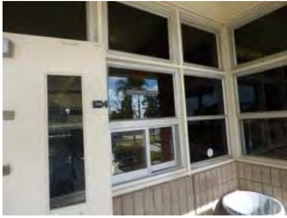
Photo #7: Office entry
