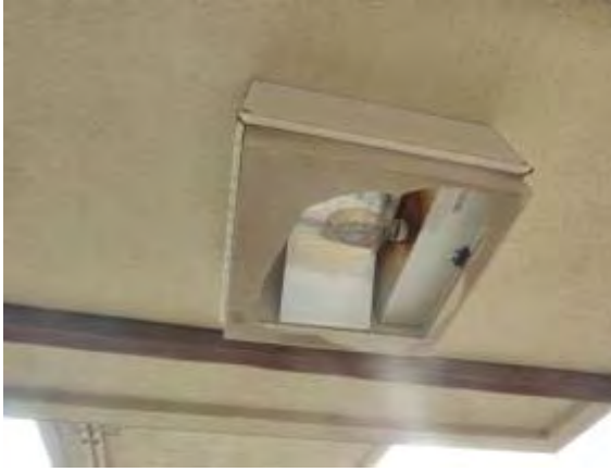
Photo #37: Damaged soffit lighting at walkway roof
