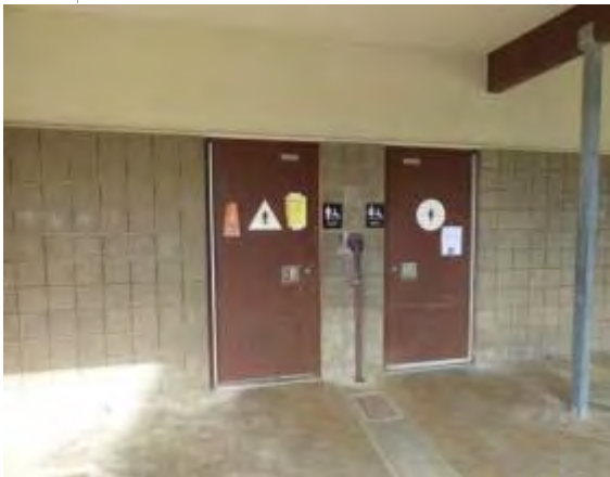
Photo #39: Service doors at student restroom
