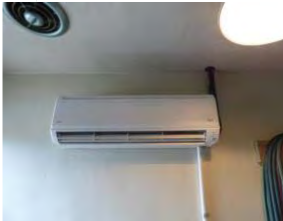
Photo #45: HVAC split system at office server room
