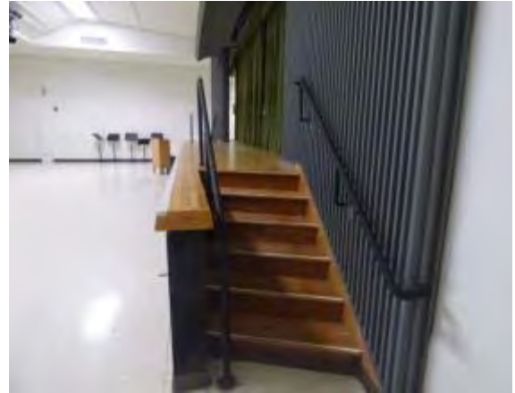
Photo #14: Multi-purpose building stage stair
