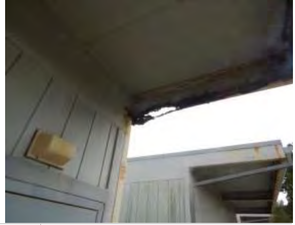
Photo #50: Damages at portable classroom roof edge
