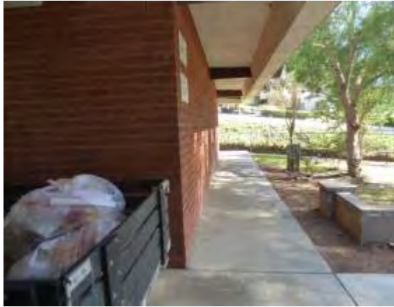
Photo #25: Walkway around classroom buildings
