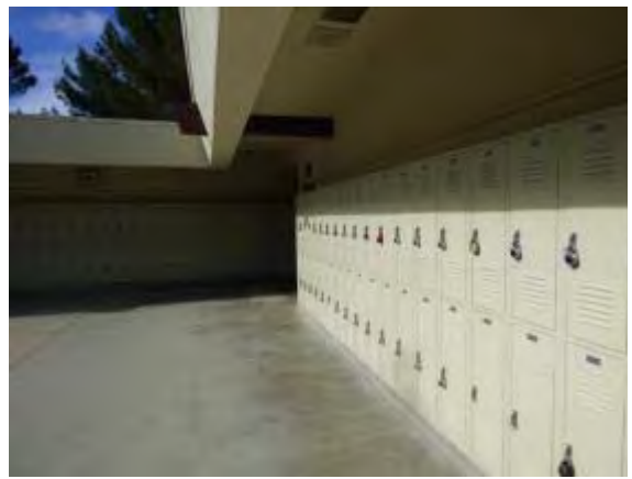
Photo #24: Student lockers at center courtyard in 3 classroom buildings #300, 400 and 500
