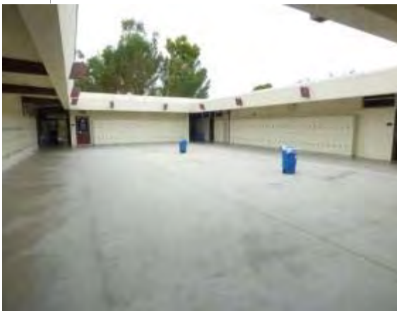
Photo #23: Center courtyard at 3 classroom buildings #300, 400 and 500
