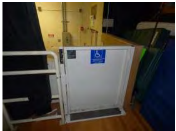
Photo #17: Multi-purpose building back stage lift
