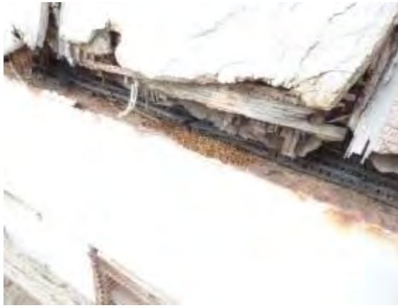
Photo #51: Damages at portable classroom wall near ground level
