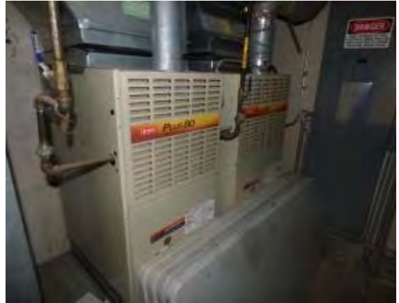
Photo #44: Forced air furnace at mechanical room
