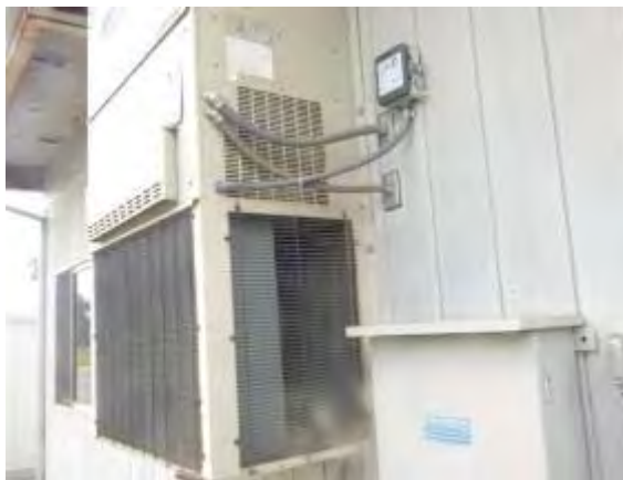
Photo #53: HVAC package unit at portable classrooms
