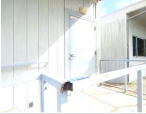
Photo #49: Damages at classroom portable building entry door and ramp
