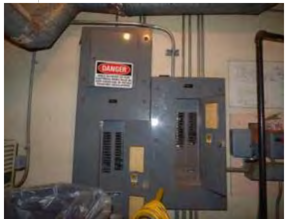
Photo #48: Electrical panels throughout buildings
