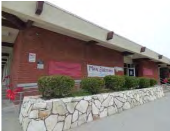
Photo #3: Close-up front exterior
