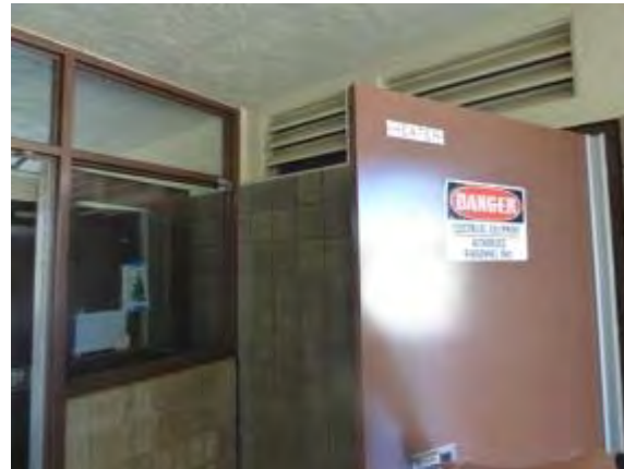
Photo #28: Classroom building mechanical room and service door
