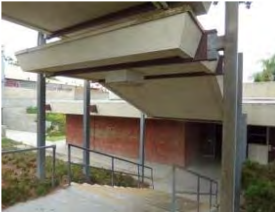
Photo #33: Stair to bldg. #300 with covered walkway
