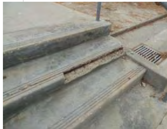
Photo #30: Damaged nosing close-up at exterior walkway stair
