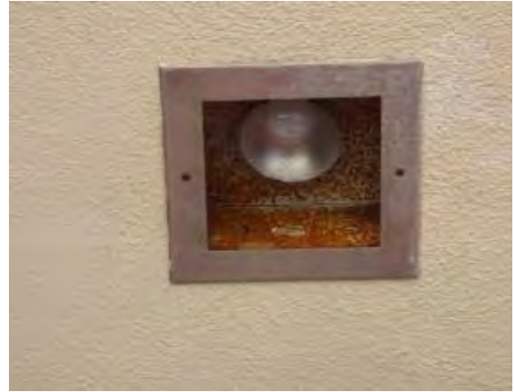
Photo #38: Corroded soffit lighting at walkway roof
