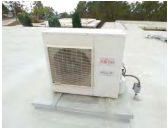
Photo #46: HVAC split system at office roof
