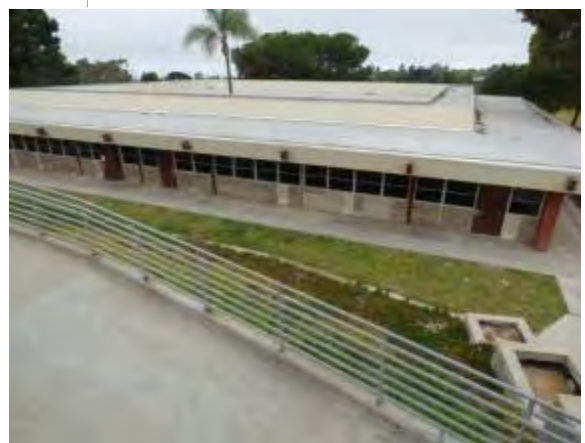
Photo #6: Classroom building exterior
