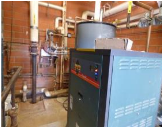
Photo #25: Boiler #2 and hot water storage tank
