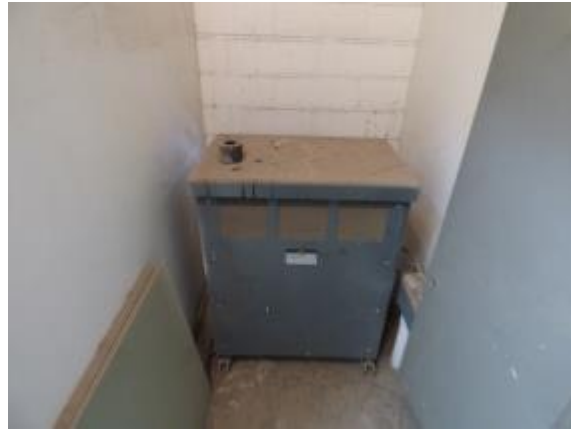
Photo #32: Step down transformer
