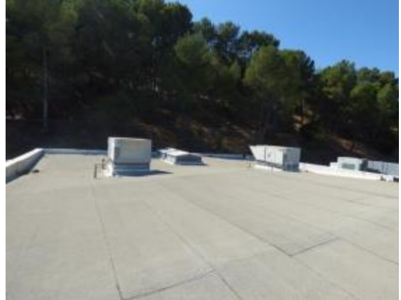
Photo #16: Modified built up roof above TAB building
