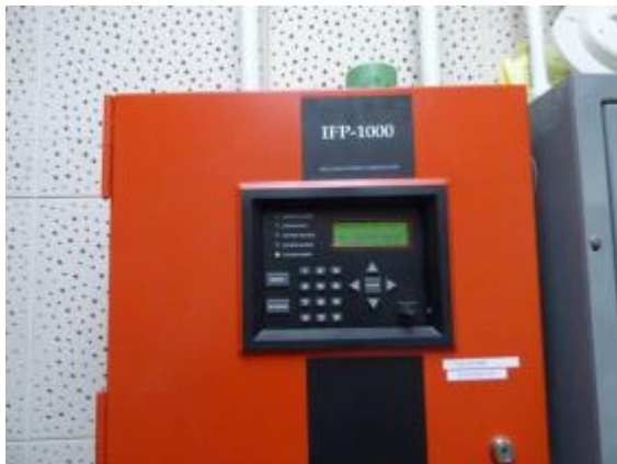
Photo #39: Fire Control Main Panel
