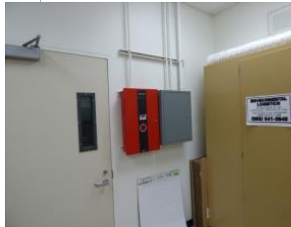
Photo #40: Fire Control Sub-Panel
