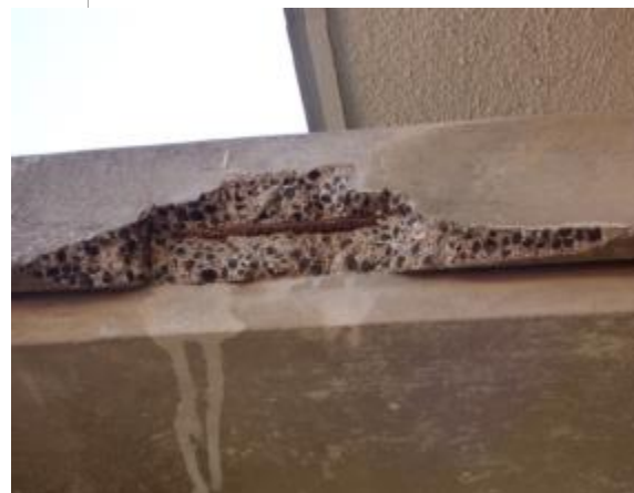
Photo #54: Concrete damage at shade structures
