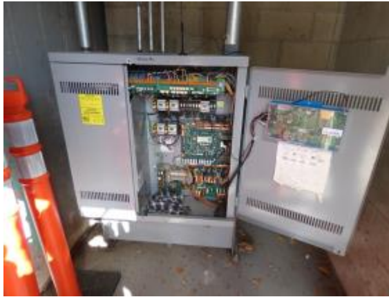
Photo #37: Elevator control
