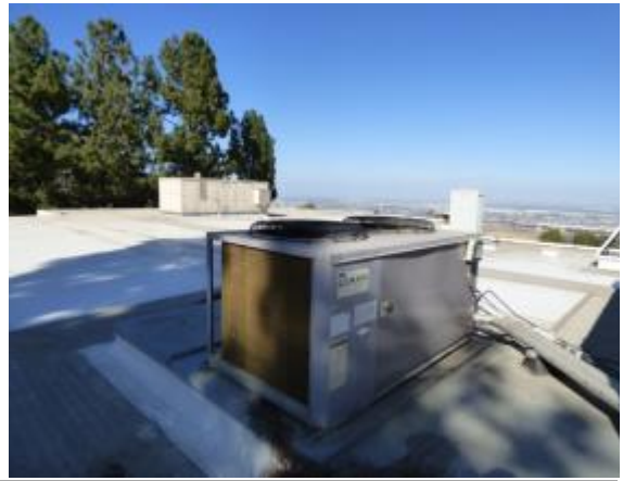
Photo #20: Roof top mechanical condenser equipment
